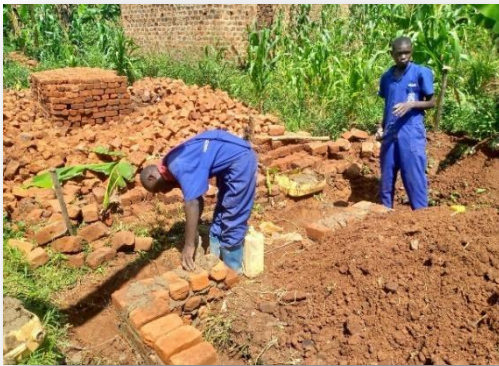
BCP learners constructing a shop for a Community member in Makukuba.
