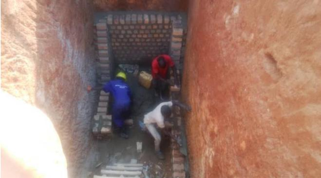
Picture above shows Building and construction Practice students constructing a septic tank at the new construction site at shared love.
