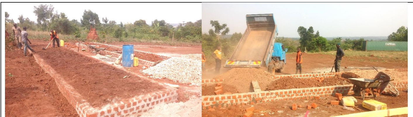
Construction of concrete Foundation Base
