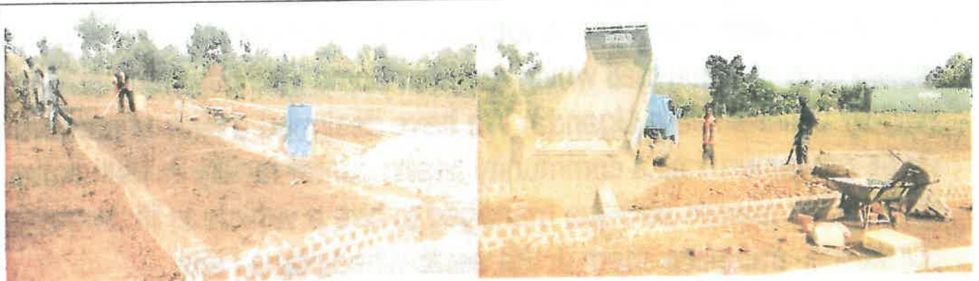
Construction of concrete Foundation Base
