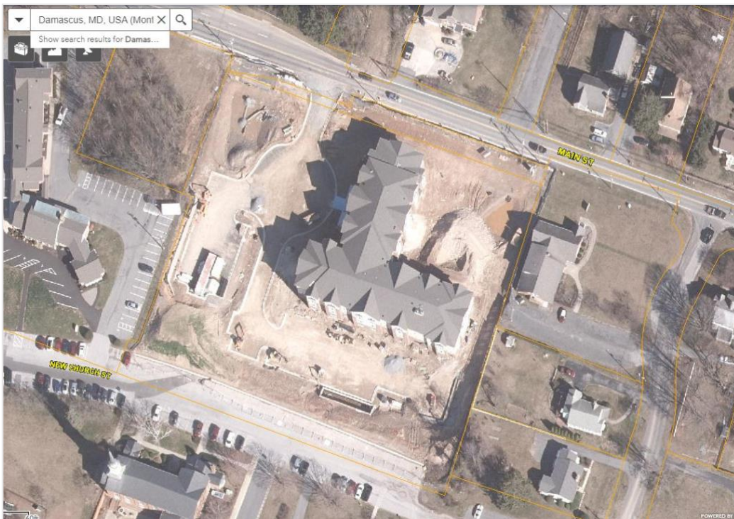
Figure 3: Victory Haven senior apartments (under construction) in Damascus; zoned CRT-1.0 C-0.5 R-0.5 H-55 T.
