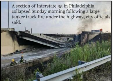
The proximate cause was a tanker truck fire that ignited on Cottman Avenue where it passes beneath the I95 roadway. The intensity and duration of the fire weakened the steel supporting beams for the overpass to the point that they could no longer support the northbound portion of the roadway.
