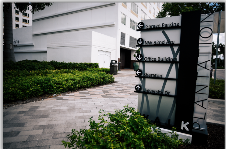
Permeable pavers installed at Plantation Walk.
