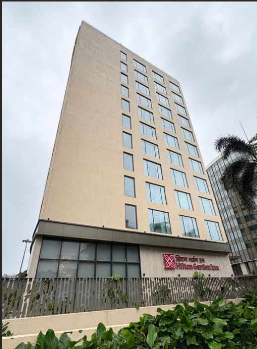
HILTON GARDEN INN, ANDHERI Seamless double-height cap curtain wall glazing designed to maximise natural light in hotel common areas. (Outside View)
