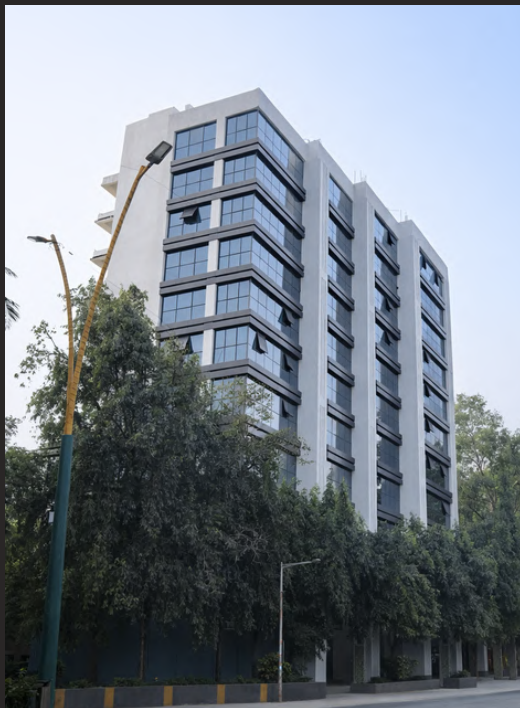
THANE BIZZ PARK, THANE Semi-united glazing with performance glass for efficiency and durability.
