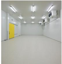
**Harvest Panels** are Insulated Metal Panels composed of steel skins laminated to a minimum of 1.6-inch ploy-isocyanurate foam core (min 2.3 pcf density).
