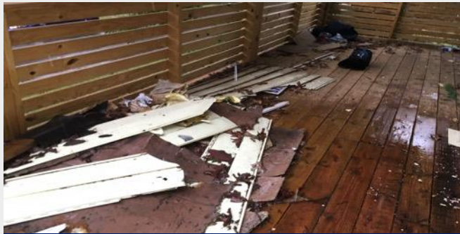
Trash and debris
