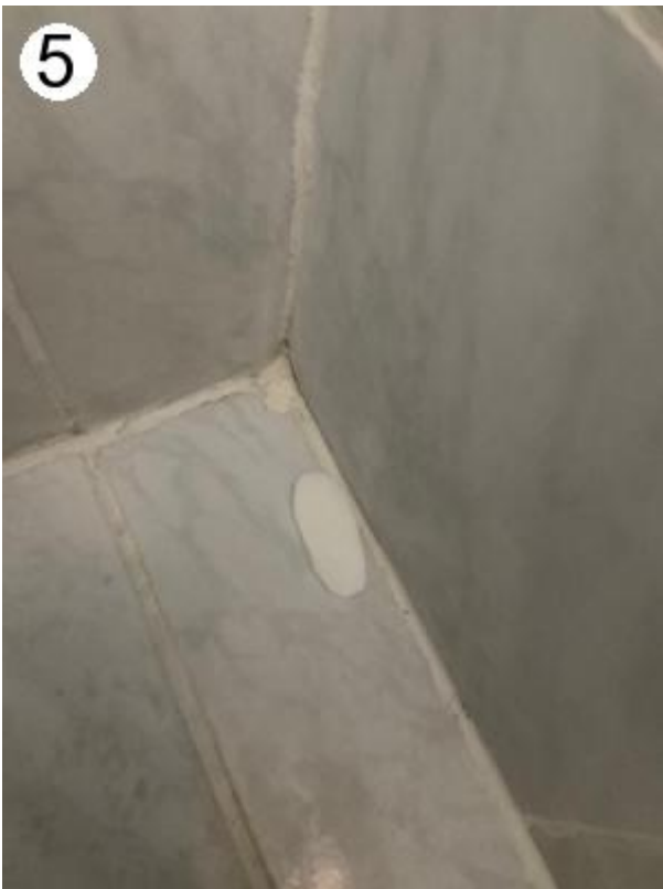
#5. Showing example of the sealant
