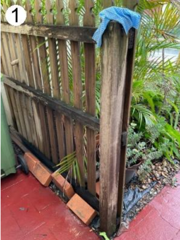
#1. Showing example of the rot
