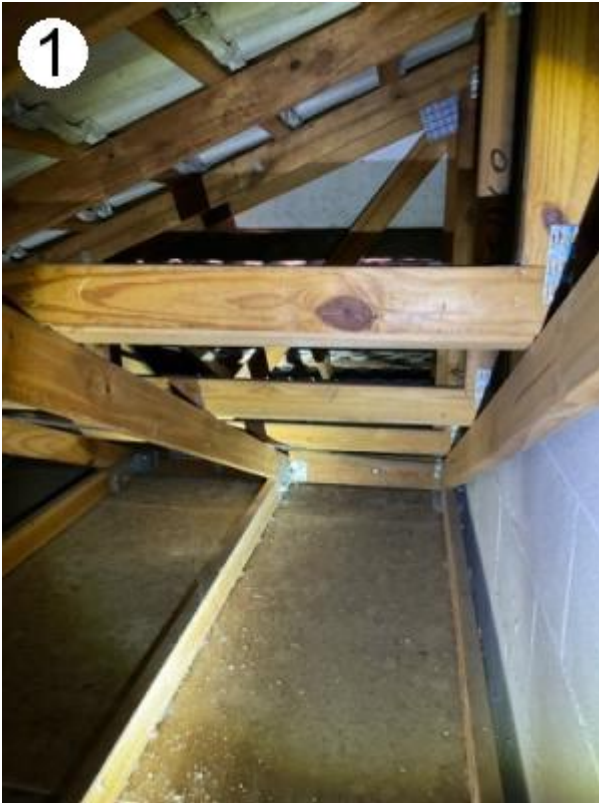
#1. Showing example of roof space height restrictions
