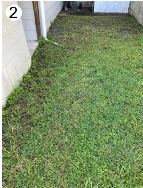
#2. Showing example of poor surface drainage
