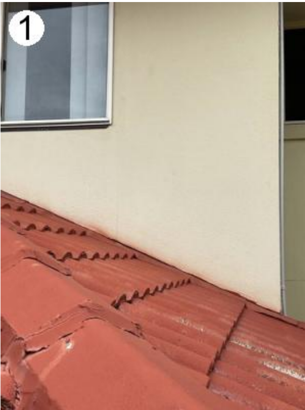
#1. Showing example of the cladding
