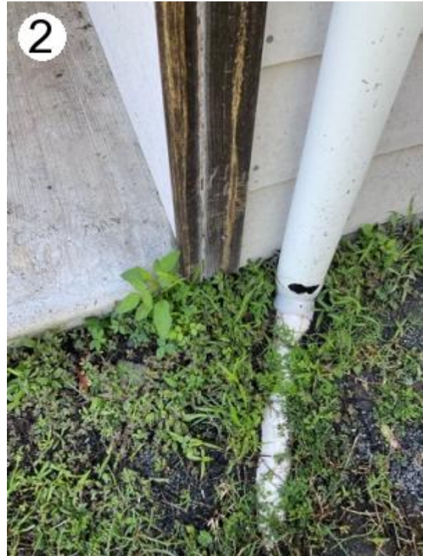
#2. Showing example of the timbers
