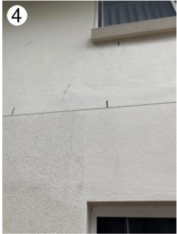
#4. Showing example of the brickwork
