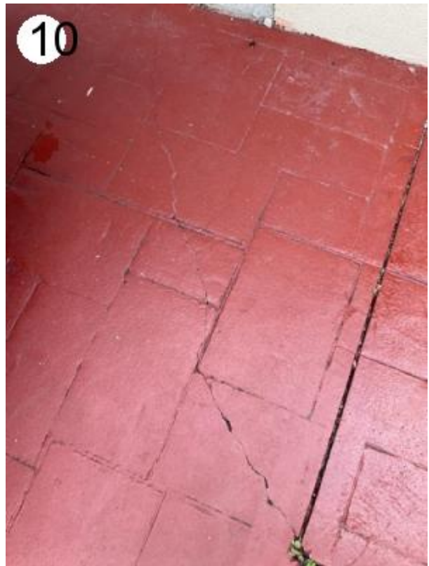
#10. Showing example of the concrete
