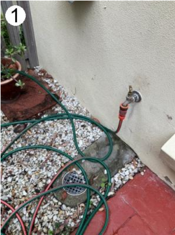
#1. Showing example of the brickwork
