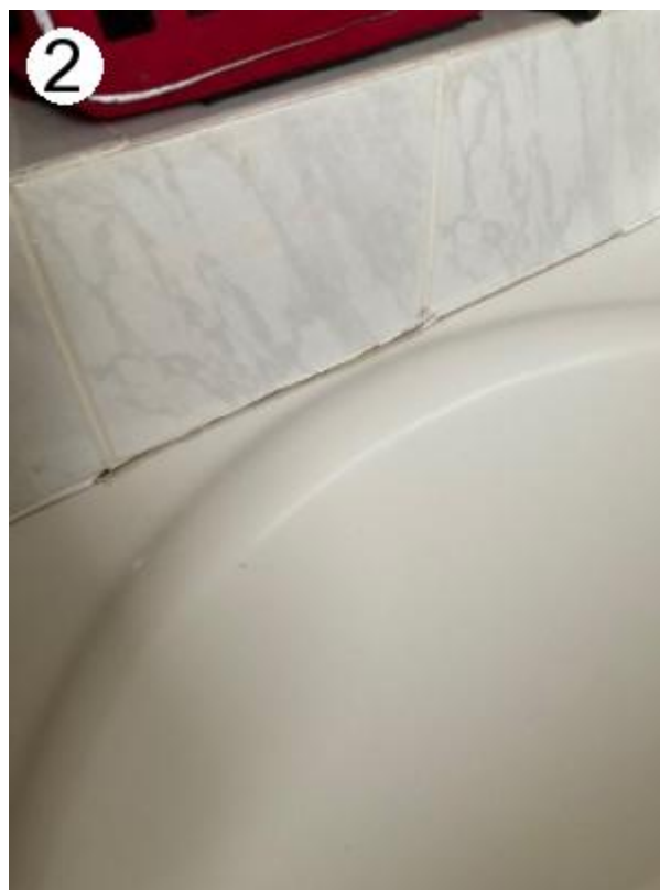
#2. Showing example of the sealant
