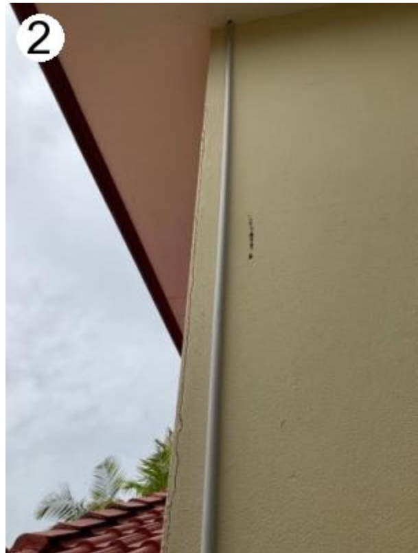
#2. Showing example of the cladding
