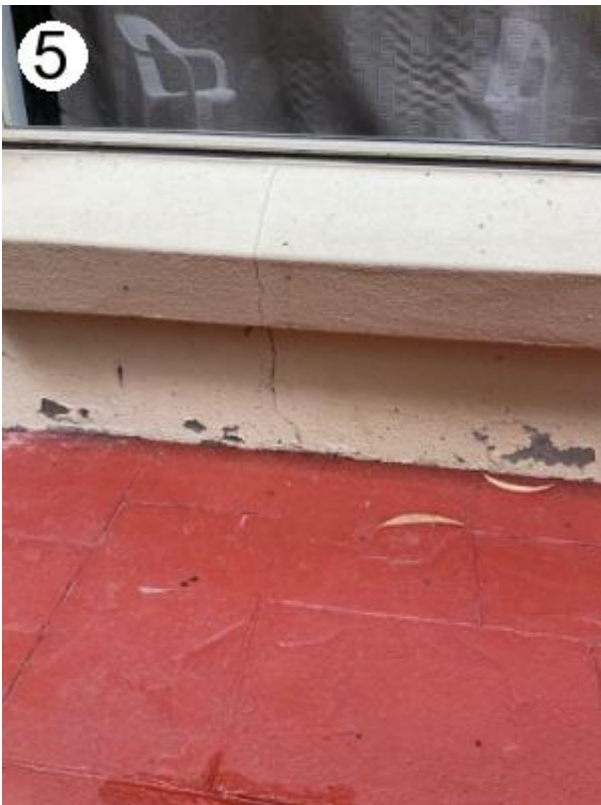
#5. Showing example of the brickwork
