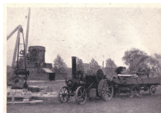
ERECTING THE FOUNTAIN IN VICTORIA PARK, ASHFORD.
