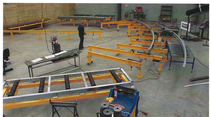
An in-house, purpose built test bed replicates the actual assembly method used on-site. Final radius measurements are made and re-checked using sophisticated laser measuring equipment to achieve an accuracy within \pm 1.5 mm of specification.
