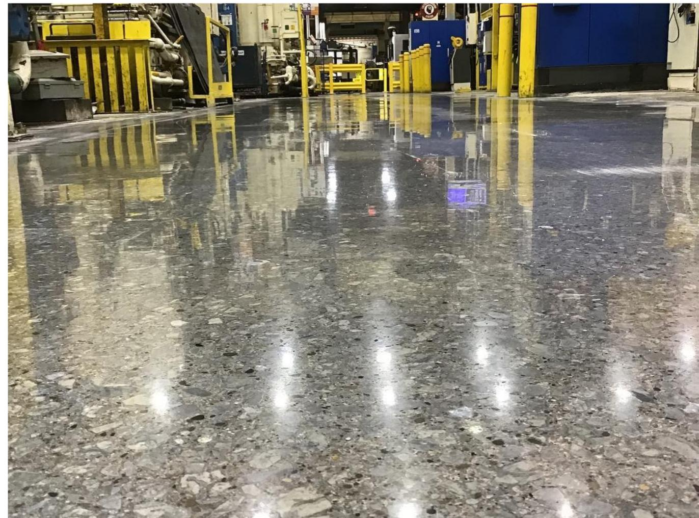
Ending the cycle of epoxy coatings at the world's largest die cast plant was paramount to saving costs to the environment and FCA's bottom line. For both new and existing slabs hydro cements were used in place of traditional admixtures and topical solutions to provide resilient floors that are easy to maintain and no longer require halting plant production to service the concrete floors.
