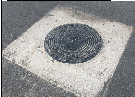
Square Concrete Support
