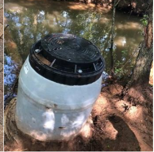
Elevated to Avoid High Water Inflow
