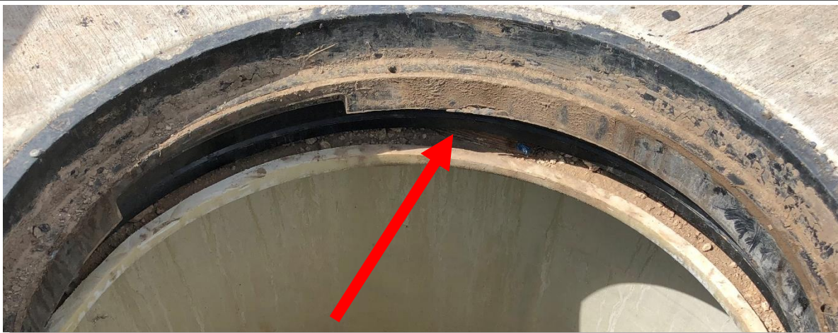
Photo Shows a Riser Ring with a Larger Clear Opening than the Frame Clear Opening
