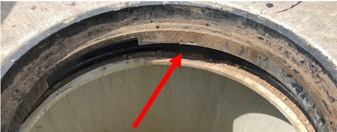
Photo Shows a Riser Ring with a Larger Clear Opening than the Frame Clear Opening
