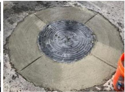
Note: Off-road some will simply backfill with dirt, raise with concrete to avoid lawnmower impact, or raise several feet to prevent water inflow.
