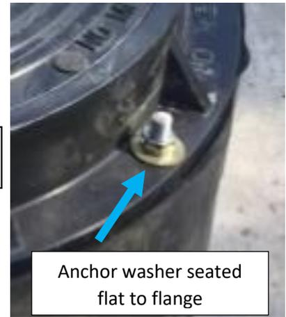
CAP frame flanges are perpendicular to the vertical frame wall. This allows for a washer to sit flat under the nut on the threaded rod used for anchoring the assembly. Non-perpendicular (radiused) flange-wall junctions can tilt the washer with one side propped up on the vertical wall joint.
