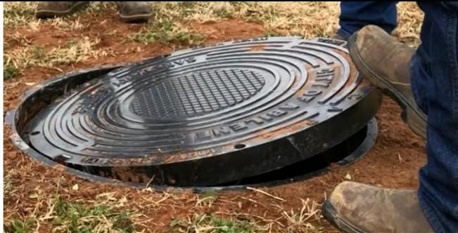
You may need to rotate the cover if the holes and hardware do not line up. The frame has shapes (triangles, stars) that indicate where the bolt holes should be aligned to have the cover and frame holes centered on each other. The frame also has indicators for paddle lock notches.
