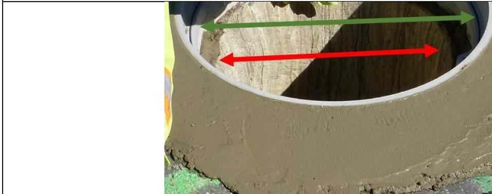
3) You may need to cut into the concrete or asphalt with a jackhammer, pick, or saw. Remove the current cover and frame. The old cover and frame may be very heavy depending on the size. You may need some help or tools to move it safely. Always bend knees when lifting.
