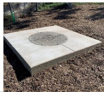
Note: If tripod use is planned for entering and exiting the manhole, it is advisable to have a solid supporting surface large enough for the tripod base. Tripods may not be secure on dirt or soft ground. Some municipalities specify 12 feet by 12 feet of concrete around manholes.
