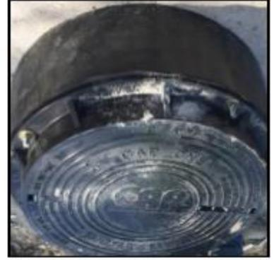
1. Mark holes in the ground using the frame anchor holes as the template. Insert anchors (e.g. Redhead) at the anchor hole locations. Attach threaded rods.
