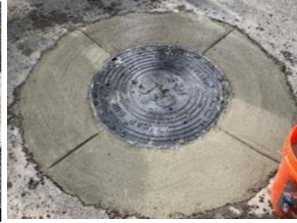
Circle with Expansion Joints
