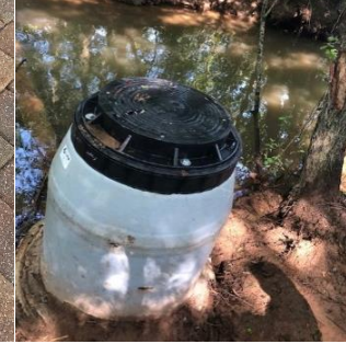
Elevated to Avoid High Water Inflow
