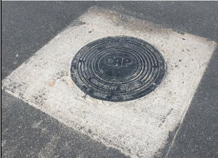
Square Concrete Support
