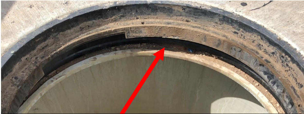
Photo Shows a Riser Ring with a Larger Clear Opening than the Frame Clear Opening
