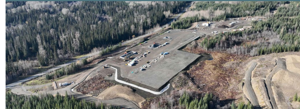
BC Hydro's Treaty Creek Terminal
