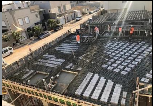
Construction works (Blacksmithing and carpentry)
