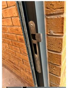
50mm rebate post with 10mm slam stip. Fixing type to wall.
