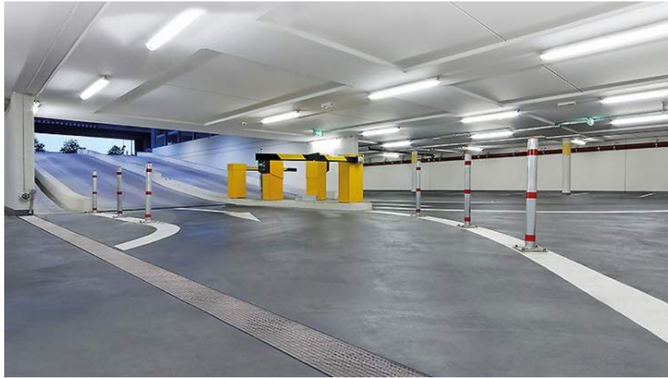
Figure 14: Parking Garage Trench Drain
