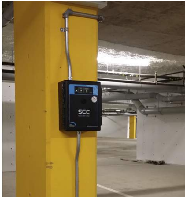
Figure 7: Toxic and Combustible Gas Detector
