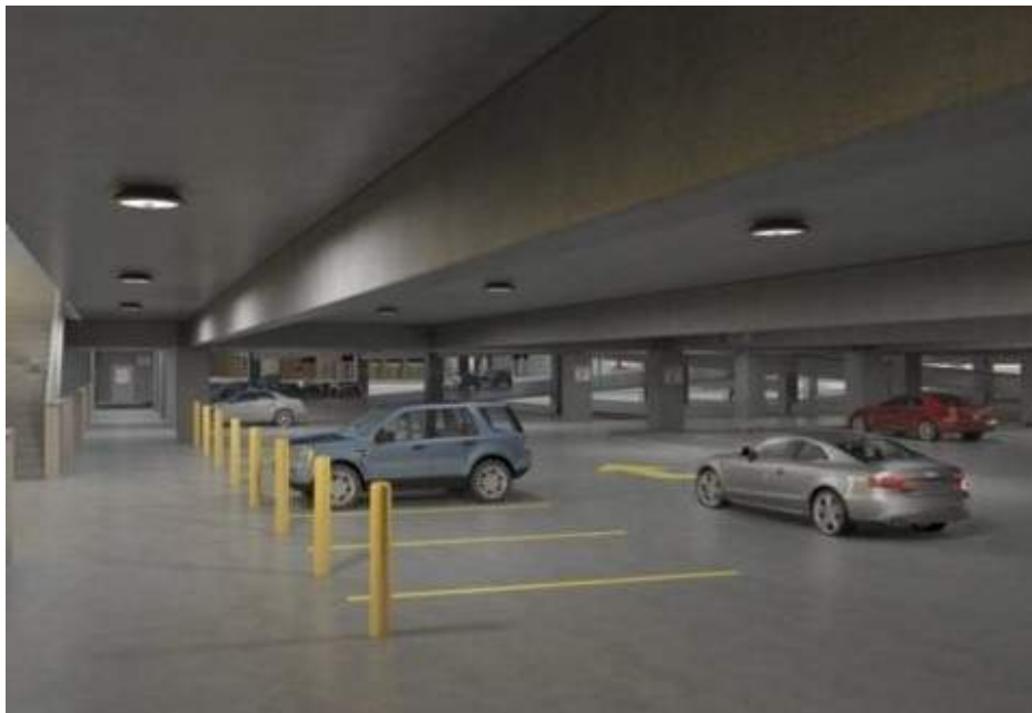
Figure 19: Energy Efficient Lighting System
