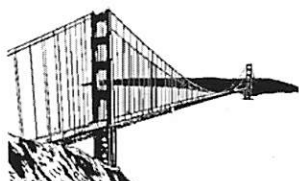
Golden Gate Bridge
