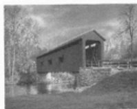
Pass Through Covered Bridge
