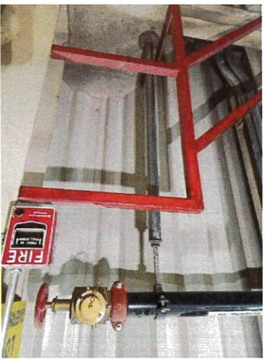
3 rd Floor – top of stairs
