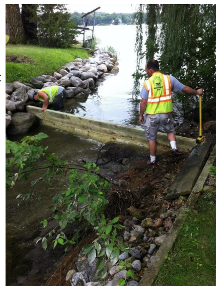
Workers installing dam between Spring Lake and Upper Prior Lake in July 2014.
