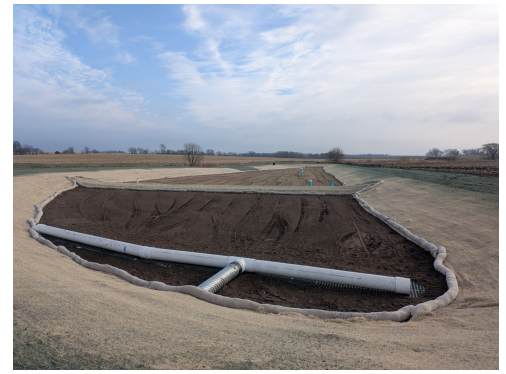
The Swamp Lake Iron-Enhanced Sand Filter will remove pollutants from water from Swamp Lake, including the nutrient phosphorus, which feeds algae. Swamp Lake is in Sand Creek Township and drains to Spring Lake through County Ditch 13.
