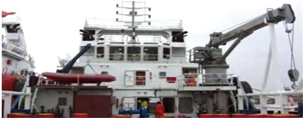
Installation of Deck Equipment on an Anchor Handling Tug Supply Vessel
