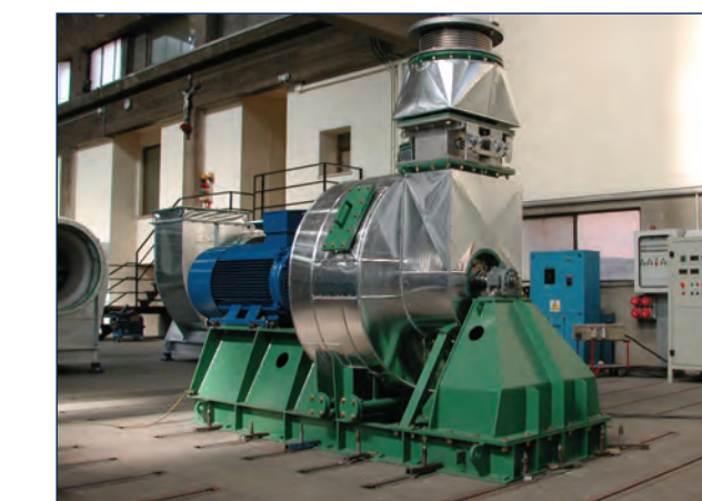
◆ COKE OVEN GAS BLOWER
