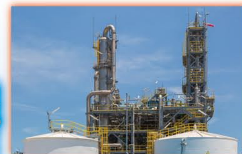
Oil Refinery Plant
