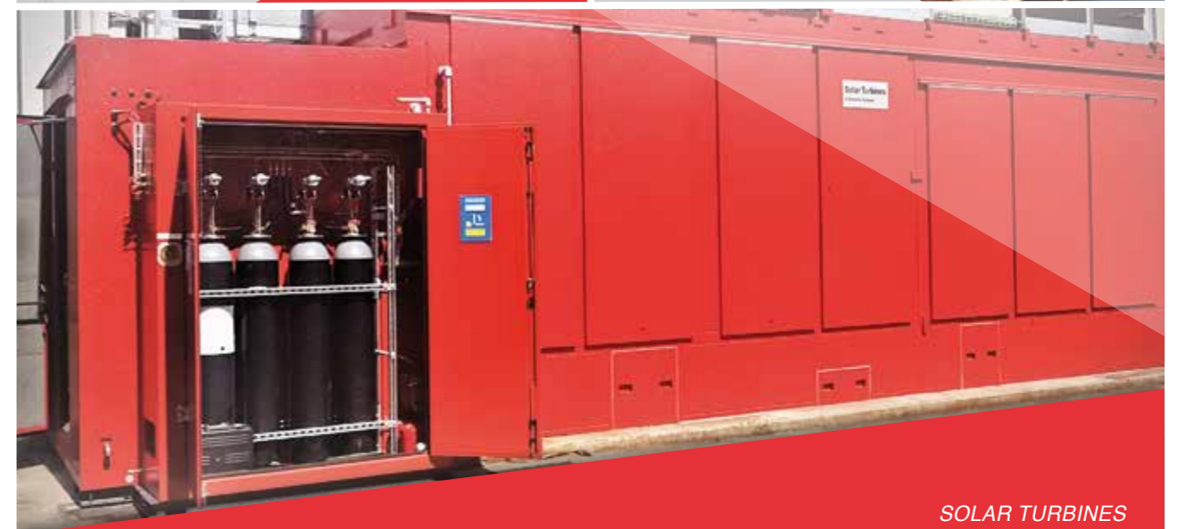
DATA CENTER FOUR Novec 1230 fire protection system
