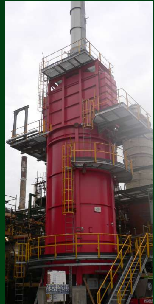
Full Replacement of an existing Fired Heater
