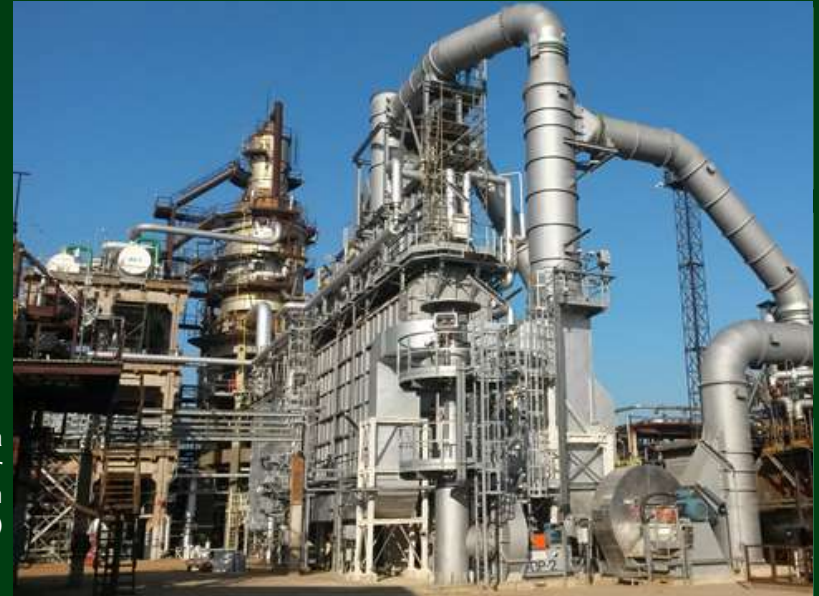
ORLEN REFINERY, Lithuania Visbreaker Vacuum Heater with APH system (21 MW)
