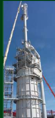
Neste Oil Porvoo, Finland Hot Oil Heater with APH (30 MW)
