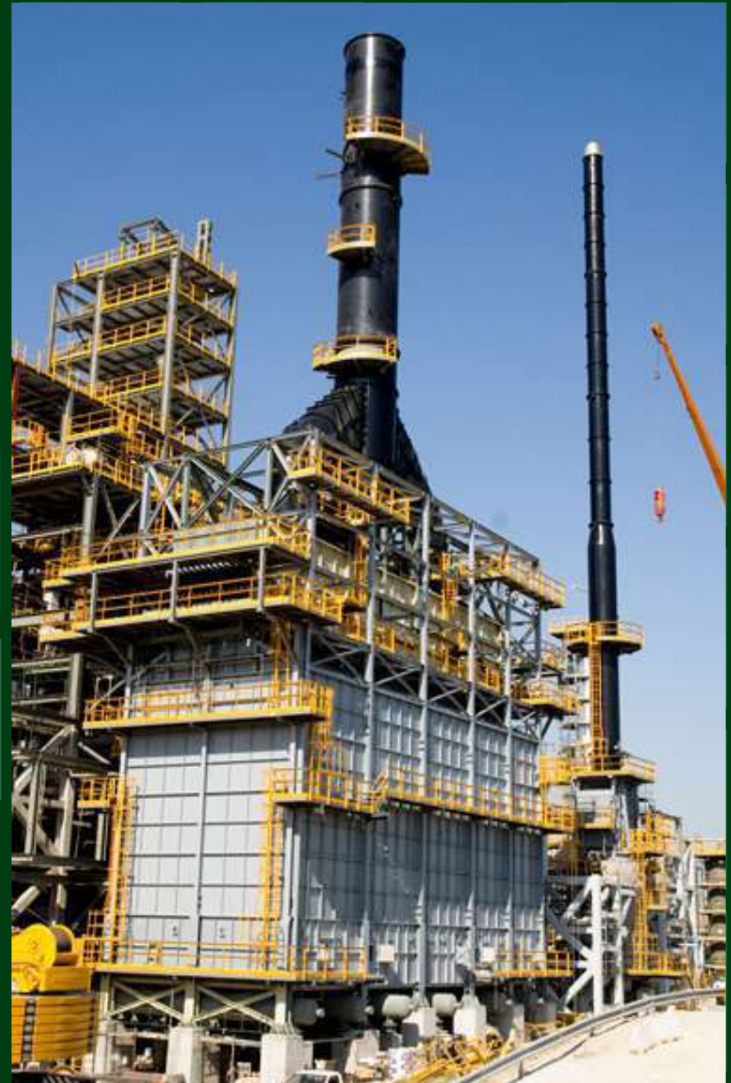
HEL.PE Refinery (former ESSO Refinery) Thessaloniki, Greece Octanizer Heater box type with three cells and arbor coils (47 MW) and Stabilizer Reboiler (6 MW)
