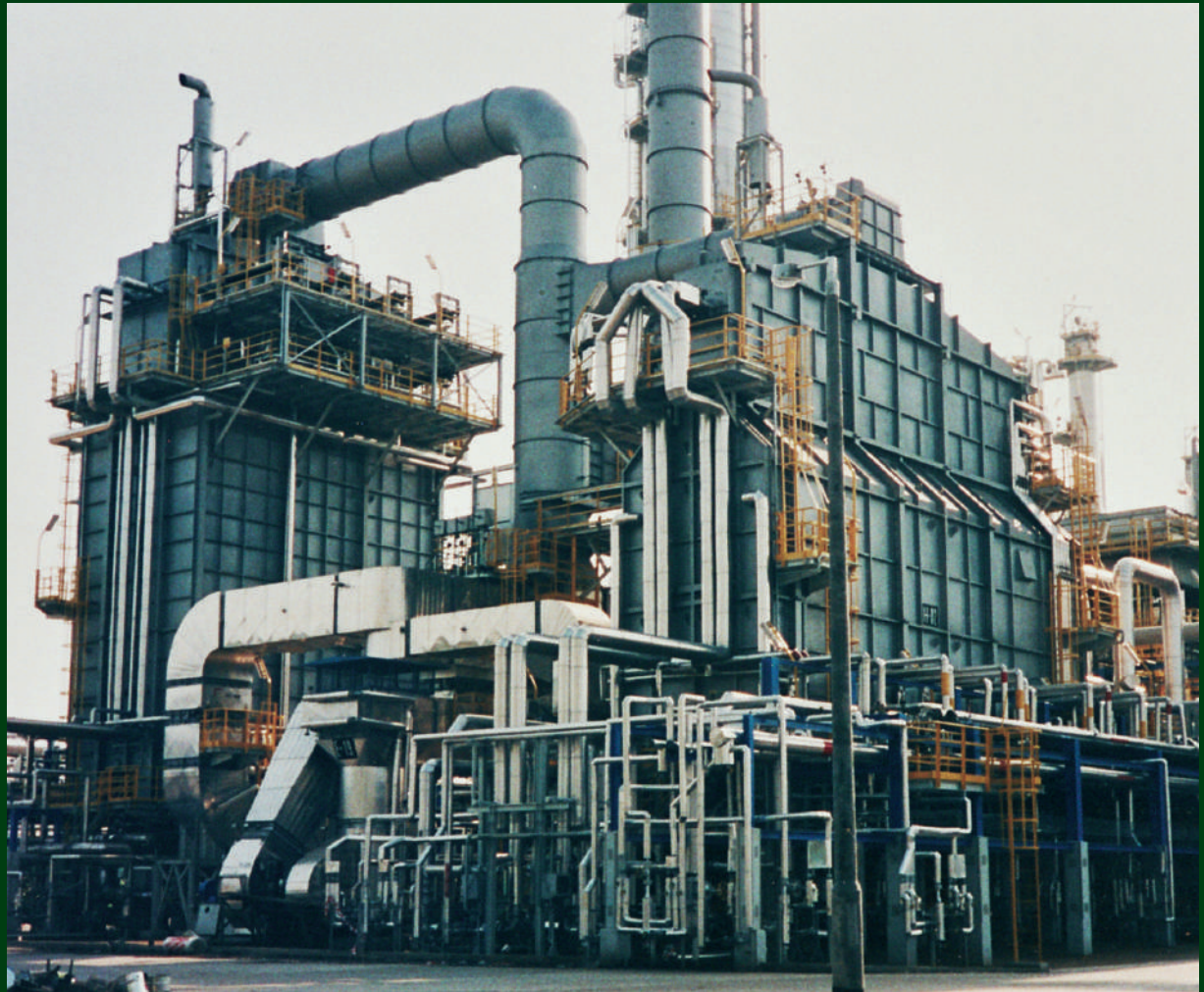
PKN ORLEN Plock, Poland CDP6 Heaters: Topping (40 MW) Vacuum (15 MW) with common APH
