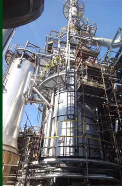
SARAS Refinery, Italy HDS Reactor Heater (8 MW) and Stabilizer Reboiler (8 MW) with APH
