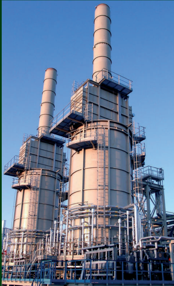
Petrofac UK for Severtex, Shapkino, Russia South Shapkino Oil Field Development Two Hot Oil Heaters (16 MW each)
