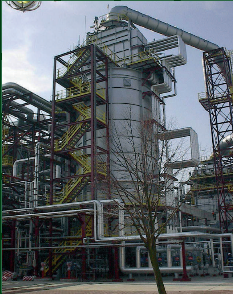
FLUOR DANIEL for PKN ORLEN, Plock, Poland CDU 3 Unit: Topping (64 MW) Vacuum (32 MW) with common APH System
