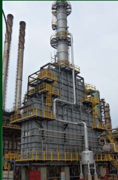
TOR Refinery, Tema, Ghana Crude Heater (28 MW)
