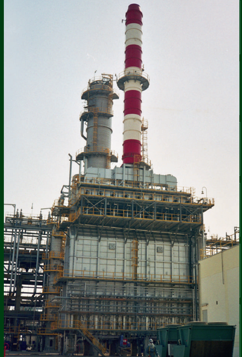
Technip for ENOC Dubai, UAE Two Topping Heaters (50 MW each)
