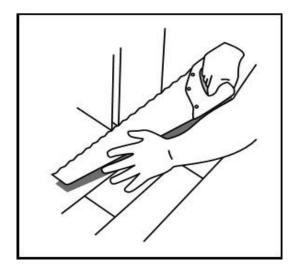
**1. Under Cut All Door Jambs and Moldings:** Remove all shoe and base moldings to ensure adequate expansion space. Use scrap piece of flooring to establish height of cut. Remember to account for height of underlayment.
