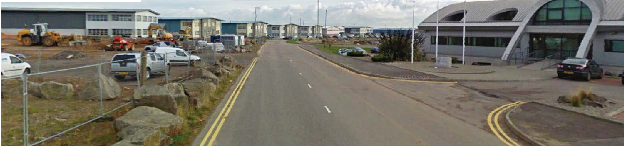
Development at Altens Industrial Estate
