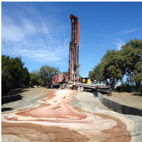
Drilling rig at BSEACD's multiport monitor well near Bee Cave
