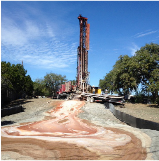
Drilling rig at the Travis County multiport monitor well
