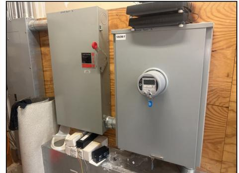
Electrical meters were located in electrical room and disconnects for each suite were located at the meter
