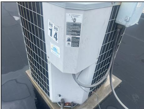
Exterior cooling unit compressor data tag was not present in unit 14.
