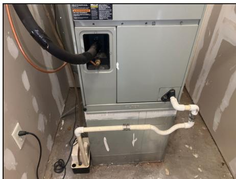
Evaporator coil portion of the cooling system in main hallway utility closet. Trane. Age 19.
