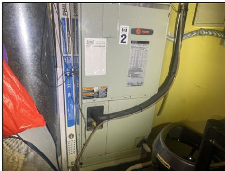
Evaporator coil portion of the cooling system in suite 120. Trane. Age 19
