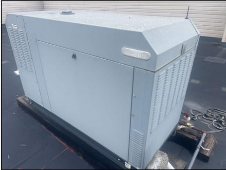
Back up generator was connected to a gas line. Gas line to roof is not in service. Generator is not available for use without gas.
