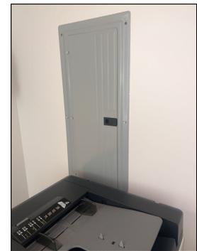
Sub panel in second floor main was obstructed. Not inspected. Sub panels should be accessible.
