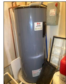
Water heater located in the second floor main suite roof access room. Rheem. Age 19. Capacity 50 gallons.
