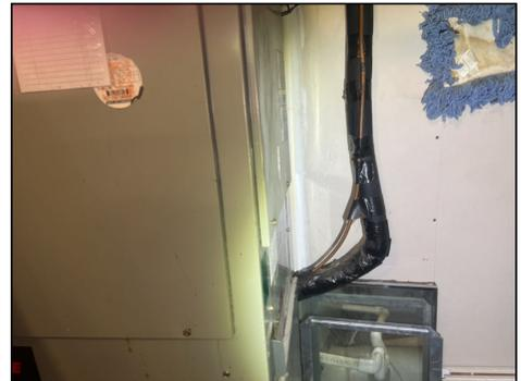
Evaporator coil portion of the cooling system in suite 130. Trane. Age 20
