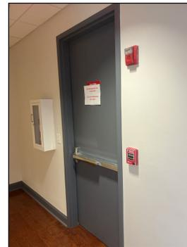
Emergency exit from second floor was connected to alarm, which would activate if opened. Not tested.
