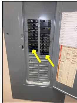
Open knockouts observed in second floor electrical room service panel cover.
