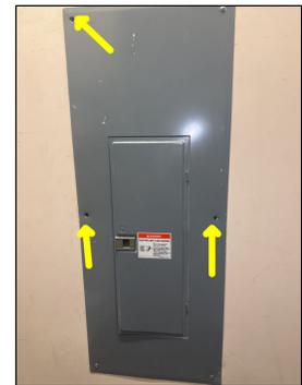
Missing screws noted at panel cover in second floor main suite electrical room.
