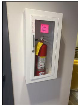
Fire extinguisher box near reception area on second floor was locked. This should be accessible in case of emergency.
