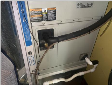
Evaporator coil portion of the cooling system in suite 120. Trane. Age 20
