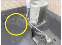
Billowing observed on roof covering adjacent to AC compressor 11.
