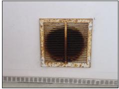
Rust observed on exterior ventilation duct covers
