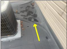
Billowing observed on roof covering. Recommend contacting a licensed roofing contractor to review repair options.
