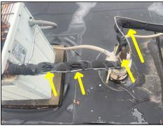
Refrigerant line insulation is damaged at one or more roof cooling compressors. Recommend repairs for improved performance.
