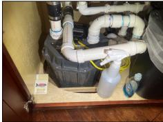
Ejector pump located under second floor break room sink. Operational at time of inspection.
