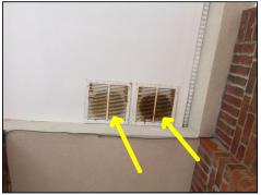
Rust observed on exterior ventilation duct covers
