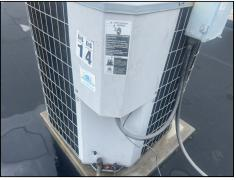
Exterior cooling unit compressor data tag was not present in unit 14.
