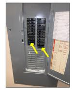
Open knockouts observed in second floor electrical room service panel cover.
