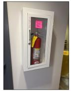
Fire extinguisher box near reception area on second floor was locked. This should be accessible in case of emergency.
