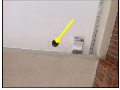
Missing exterior vent cover observed on exterior at Suite 130
