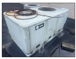
Packaged unit heating and cooling system was not operable at the time of inspection and not in use.
