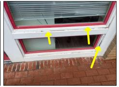
Water damaged wood trim observed at various areas on building exterior
