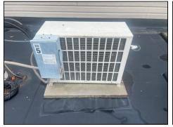
Exterior AC unit number five. Fujitsu mini split. Age unknown due to label not being legible.
