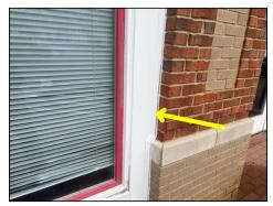
Deteriorated sealant observed at one or more areas of exterior flashing and trim.
