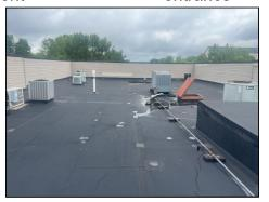
Lack of luminaire observed on rooftop. Convenience luminaire is required for maintenance on rooftop equipment.
