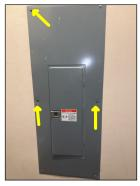
Missing screws noted at panel cover in second floor main suite electrical room.
