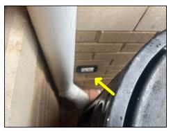
Missing/damaged weatherproof cover at left side at rear main entrance
