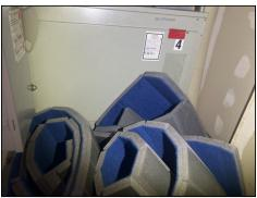
Evaporator coil portion of the cooling system in rear of suite 120 was obstructed by storage.
