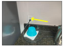
Non-GFCI outlets observed in second-floor main suite break room. GFCI's are recommended for kitchen areas.
