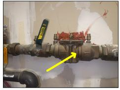
There was no visible inspection tag at the backflow preventer. Have inspected and tagged by licensed commercial plumber.
