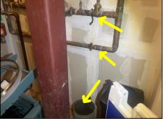
Corrosion and water, leakage, dripping from main water supply line observed
