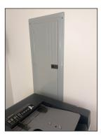
Sub panel in second floor main was obstructed. Not inspected. Sub panels should be accessible.
