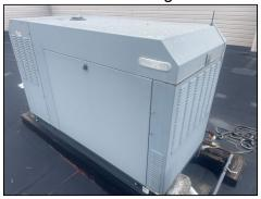
Back up generator was connected to a gas line. Gas line to roof is not in service. Generator is not available for use without gas.
