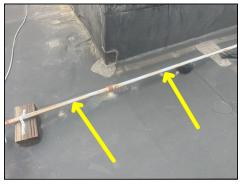
Exposed gas piping not marked for identification by a yellow label marked "Gas" in black letters occurring at intervals of 5 feet or less observed at one or more locations. See photographs for locations.
