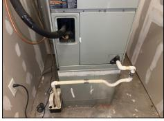
Evaporator coil portion of the cooling system in main hallway utility closet. Trane. Age 19.
