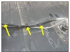
Refrigerant line insulation is damaged at one or more roof cooling compressors. Recommend repairs for improved performance.
