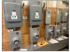
Electrical meters were located in Electrical meters were located in Electrical meters were located in electrical room and disconnects for each suite were located at the meter
