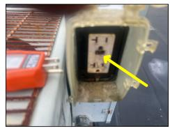
Rooftop convenience outlet was damaged. Convenience outlet are required to be GFCI and operational for repairs on rooftop equipment.
