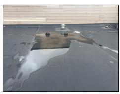
Active ponding observed on roof surface.
