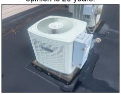
Exterior cooling unit compressor Exterior cooling unit compressor Exterior cooling unit compressor 2. Trane. Age 20.
