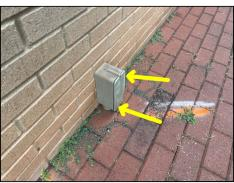
Loose screws observed that exterior electrical box at right side of building at front
