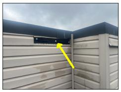
Missing section of aluminum siding, observed at Gaps observed in coping, this is a potential water rear side of parapet wall
