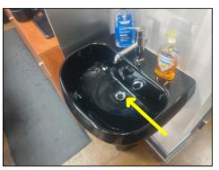
Missing drain stopper observed in hand wash sink in Suite 120
