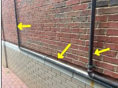
Rust observed on gas utility piping at right side
