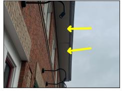
Loose soffit boards observed on rear side of building at right side
