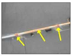
Rust observed on gas utility piping at roof
