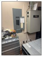
Inadequate panel access observed in second-floor data room.
