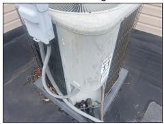
Exterior cooling unit compressor Exterior cooling unit compressor Exterior cooling unit compressor 11. Lennox. Estimated age based on professional opinion is 20 years
