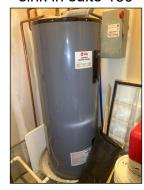
Water heater located in the second floor main suite roof access room. Rheem. Age 19. Capacity 50 gallons.
