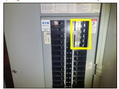
Open knockouts observed in main electrical room secondary service panel covers.
