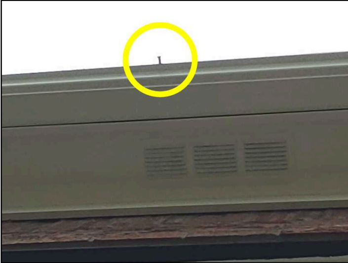
Loose gutter pins noted sporadic around home
