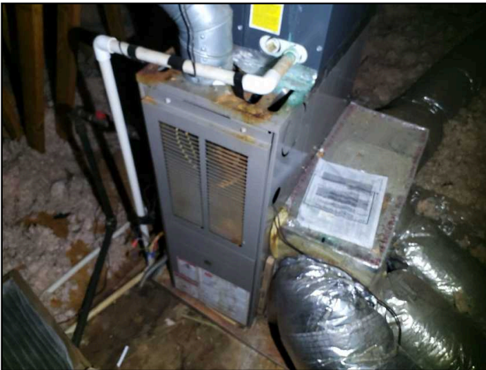
Gas furnace portion of HVAC system in attic space. unit is beyond its normal life expectancy
