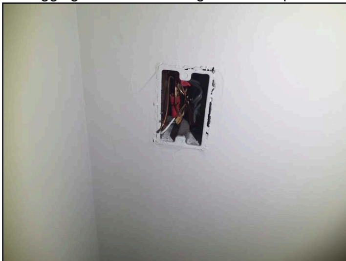
Much of the wiring appears to not be a professional installation in the basement with sagging wires and floating electrical splices.
