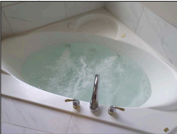
Jetted tub filled and briefly tested
