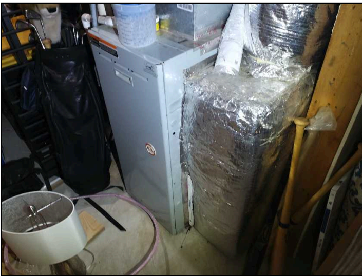
Gas furnace portion of basement HVAC system pain 1999 unit has reached its normal life expectancy
