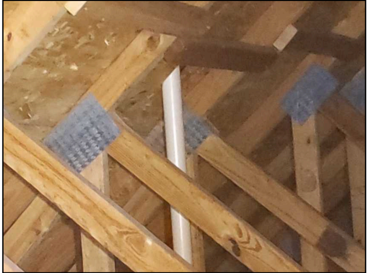
Underside of roof penetrations in attic
