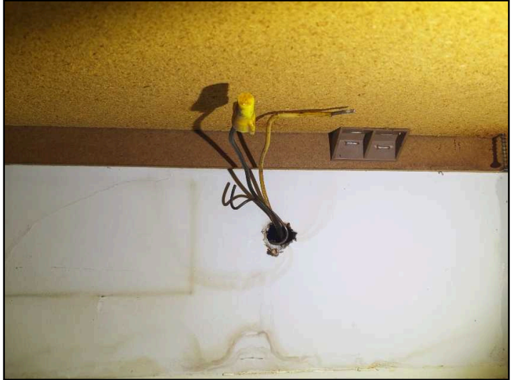
Exposed electrical wire in basement kitchen where exhaust fan should be installed
