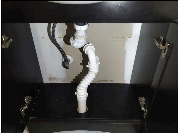
corrugated drain line with missing P-trap was noted at basement bathroom sink. These are subject to frequent clogging and should be replaced with a smooth wall pipe.
