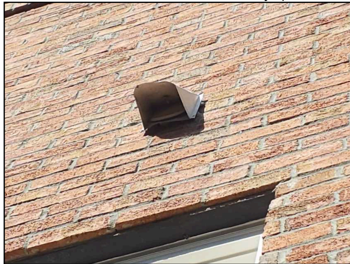
High efficiency furnace exhaust intake on right side of home should not be in close proximity to dryer exhaust vent. recommend further evaluation by qualified HVAC technician
