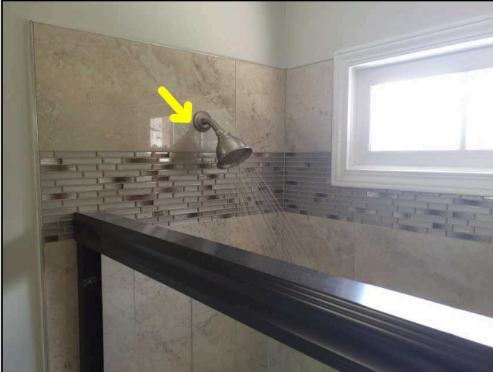
Plumbing components for main level shower head were not properly secured inside wall cavity and are extremely loose
