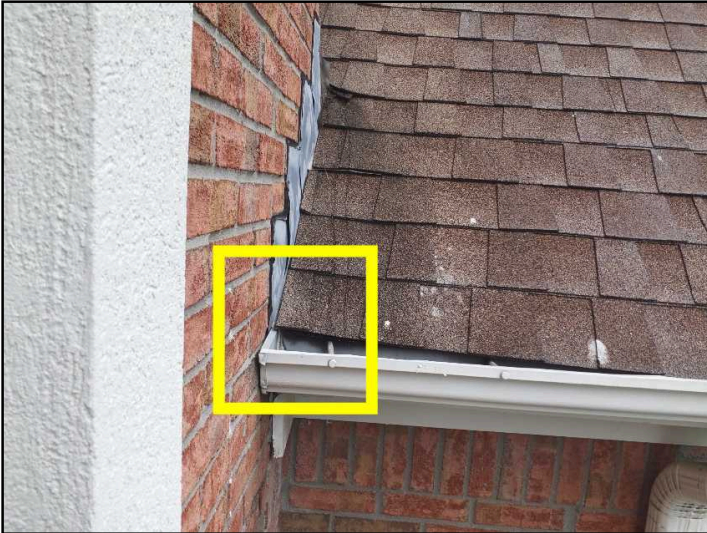
Missing kick out flashing noted at locations around the home.
