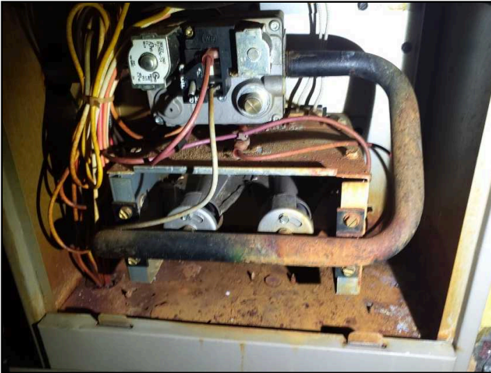
Rust noted on burners in furnace
