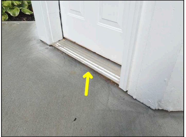
Suggested to install wood blocking beneath aluminum thresholds at exterior doors. This is to protect the threshold from any damage that may occur if stepped on.
