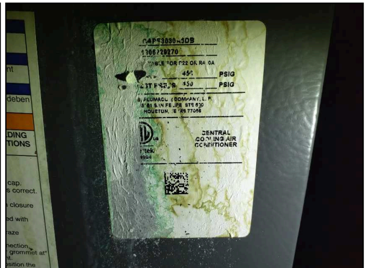
Evaporator coil data tag
