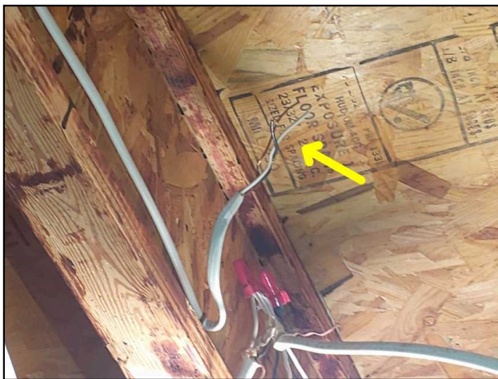
Much of the wiring appears to not be a professional installation in the basement with sagging wires and floating electrical splices.
