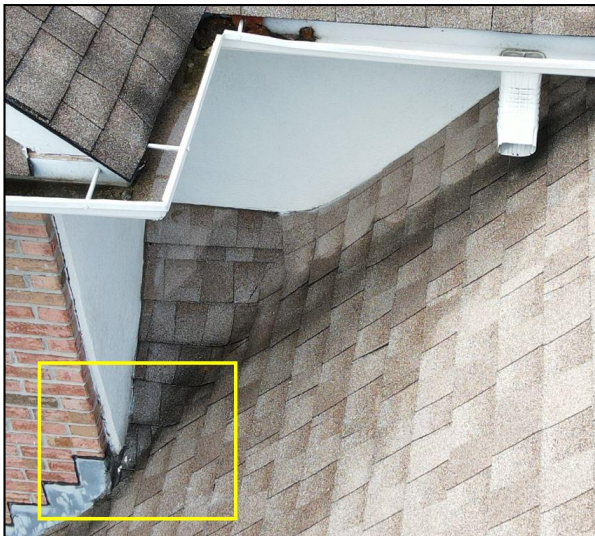
Area of roof line on right side of bay window where garage roof meets main home will have a higher potential for water intrusion due to configuration/pitch. Monitor
