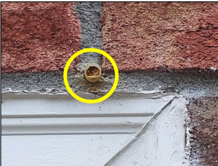
Drainage weep channels in exterior brick are clogged or missingsporadic around home. Have qualified contractor correct for proper drainage and to prevent brick from cracking.
