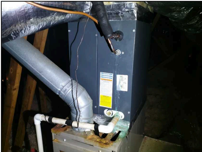
Evaporator coil portion of HVAC system in attic space 2019 Goodman
