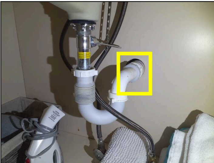
Active Plumbing Leak at sink drain on right side in master bathroom
