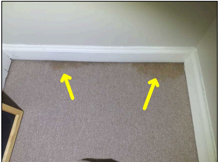
Evidence of past water event in basement around bedroom closet and bathroom.
