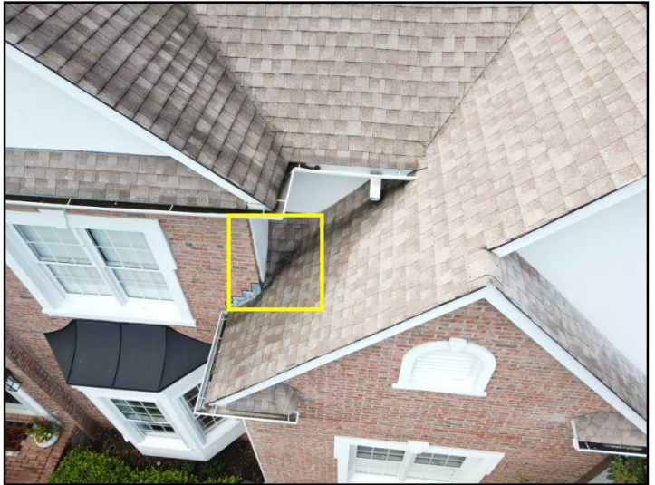
Area of roof line on right side of bay window where garage roof meets main home will have a higher potential for water intrusion due to configuration/pitch. Monitor
