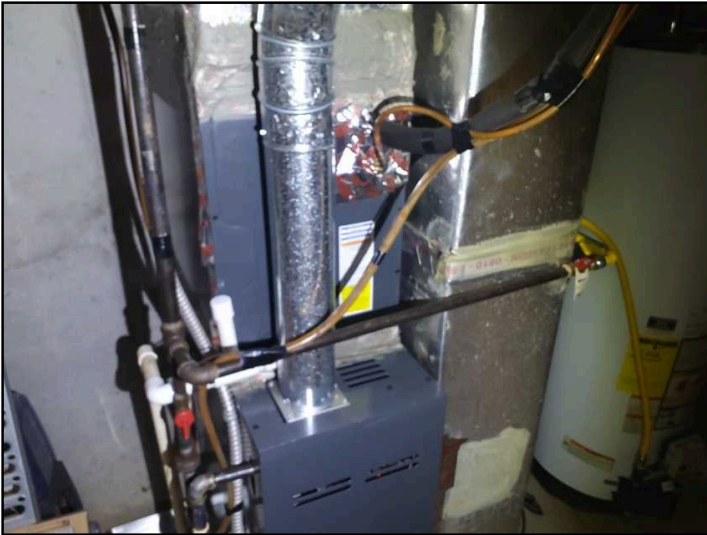
The evaporator coil portion of the HVAC system in the basement Goodman 2019
