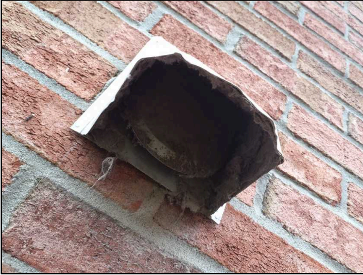
Dryer vent should be cleaned
