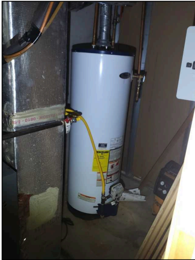
Water heater located in the basement gas Whirlpool 50 gallon 2013
