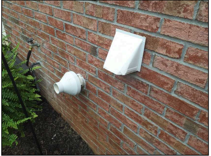
High efficiency furnace exhaust intake on right side of home should not be in close proximity to dryer exhaust vent. recommend further evaluation by qualified HVAC technician
