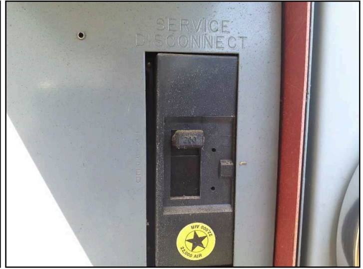
Electric meter and 200 amp shut off at the left exterior side
