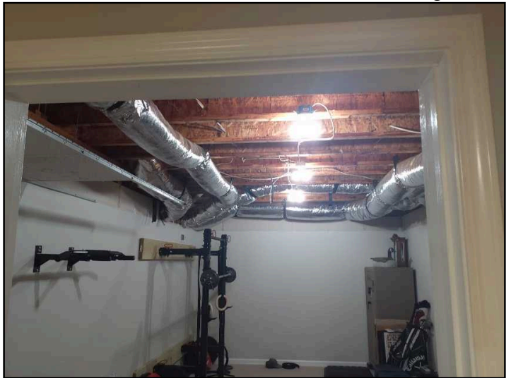
Large portion of drop ceiling is missing in area outside basement kitchen
