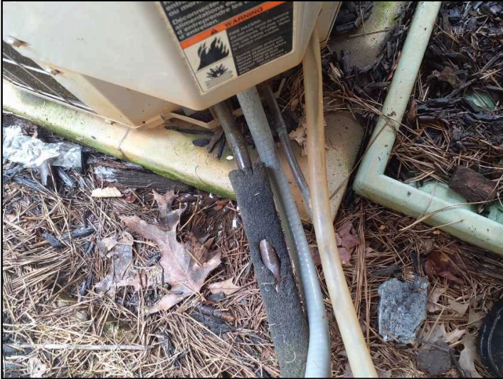
Refrigerant line insulation is damaged/missing at the outdoor ac-unit. Recommend repairs for improved performance.
