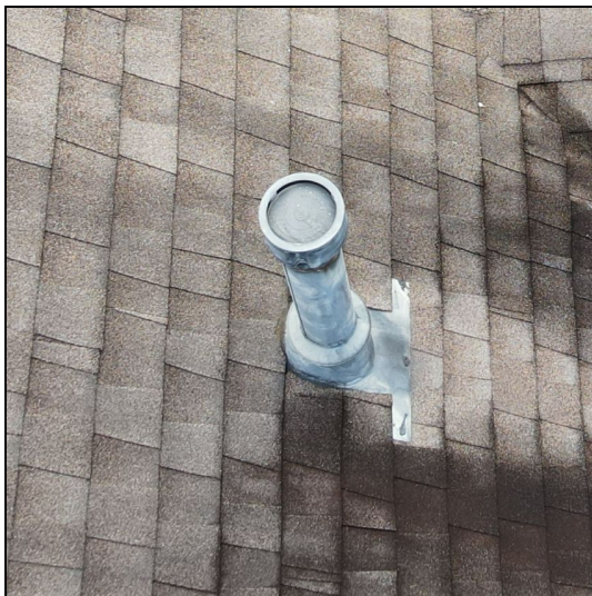
Roof penetration flashing image.
