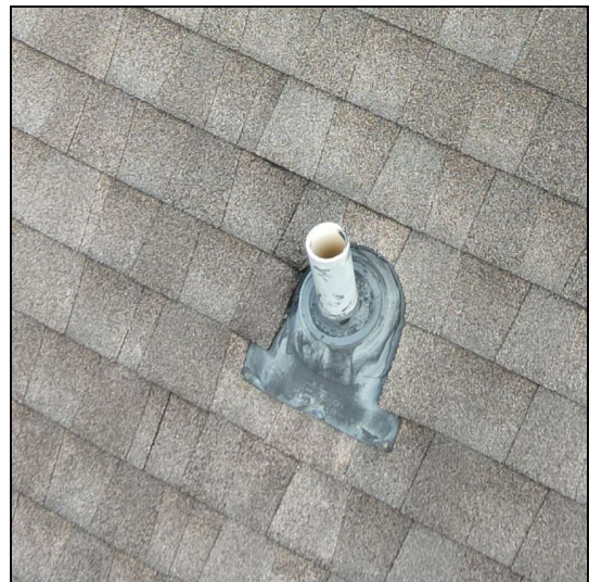
Roof penetration flashing image.
