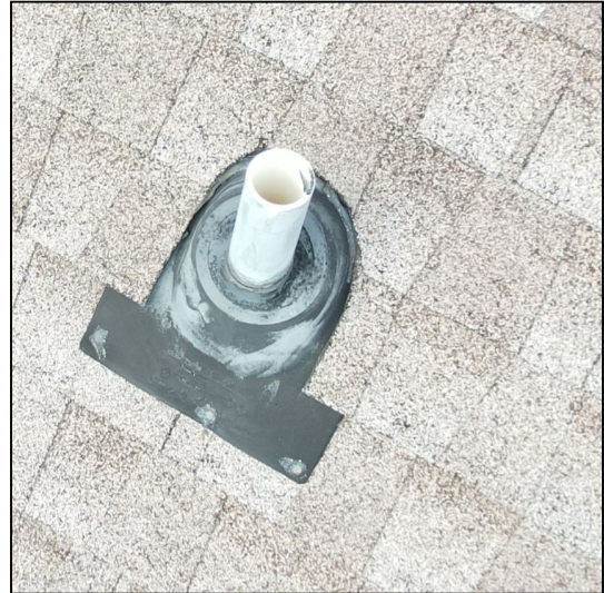
Roof penetration flashing image.
