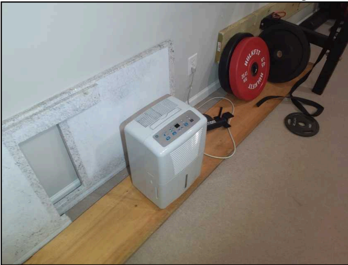
There is a dehumidifier running in the basement at the time of the inspection. This is a common way to reduce moisture in the air if the basement is not conditioned or if the AC does not run often enough.
