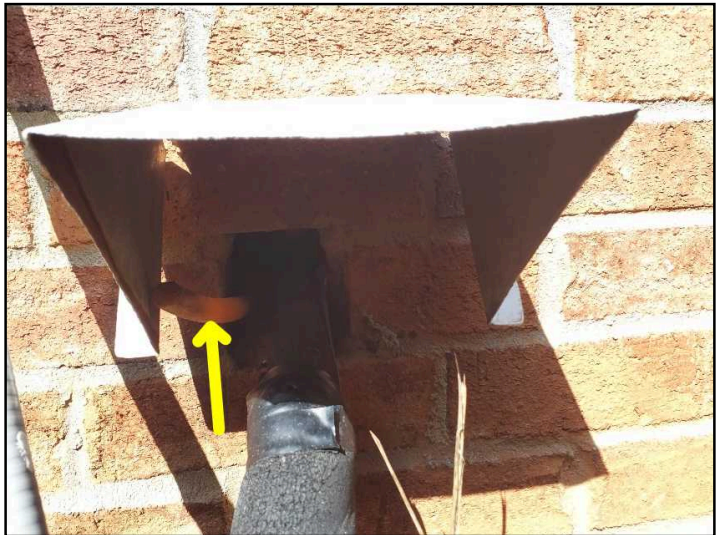
The condensate drain lines should discharge at least five feet from foundation walls to prevent water from collecting near or against the foundation walls as required by industry standards. Have a licensed HVAC or qualified contractor correct.
