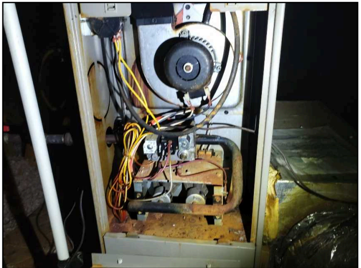
Rust noted on burners in furnace
