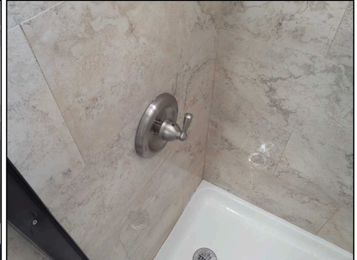
The hot and cold water lines are reversed at the shower in the main level bath room.
