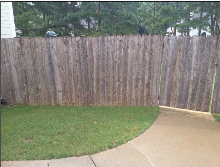
Recommend adding sealant at exterior wood fencing to extend life expectancy
