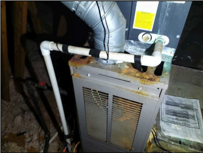
Condensation drain exiting evaporator coil is missing an access tee with a removable cap.
