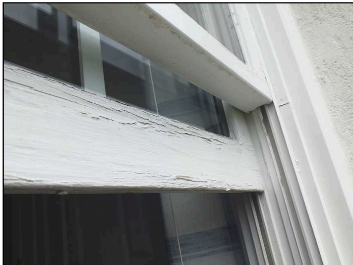
Some deterioration visible at exterior portion of windows. Recommend repair as needed to prevent deterioration
