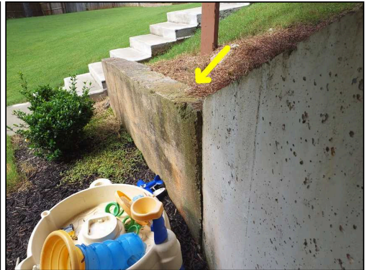
The retaining wall is leaning outward along the top below the back deck. Have a landscape contractor correct and repair as needed.
