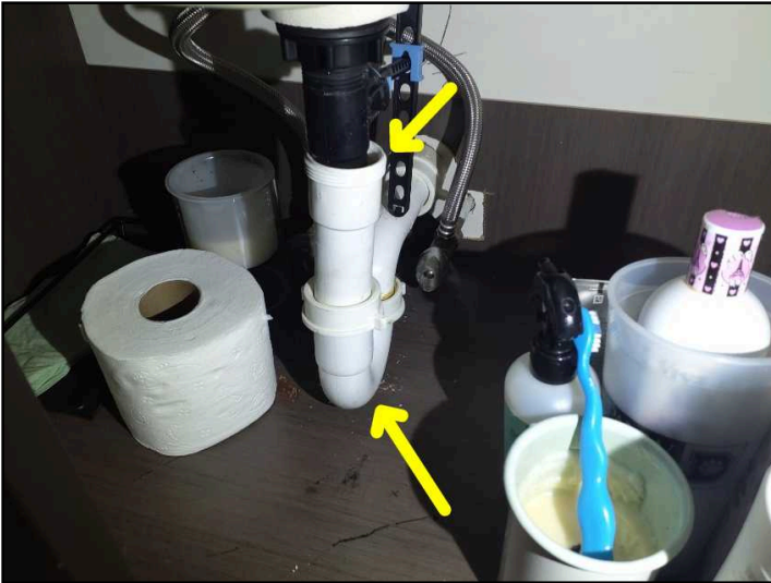
Drain below main level hall bathroom sink is not properly secured and configuration prevents removal of p-trap
