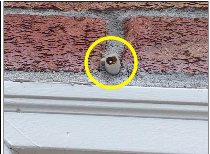
Drainage weep channels in exterior brick are clogged or missingsporadic around home. Have qualified contractor correct for proper drainage and to prevent brick from cracking.
