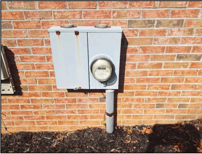
Electric meter and 200 amp shut off at the left exterior side
