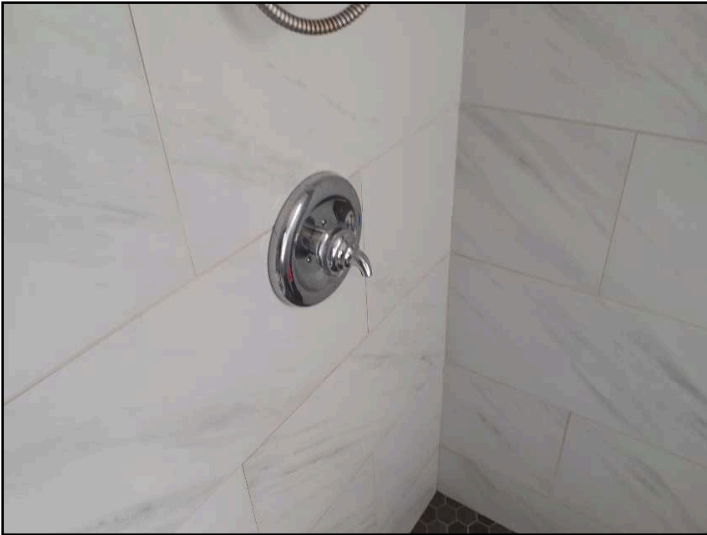
Missing or broken control handle at master shower stall
