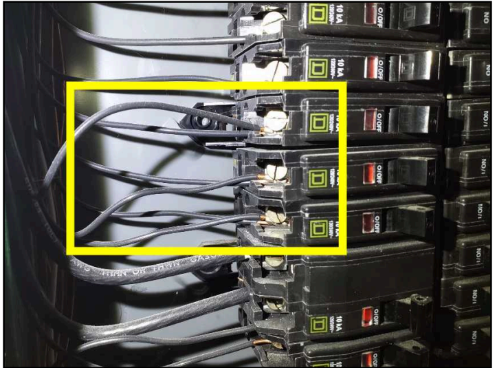
Double tapped breakers
