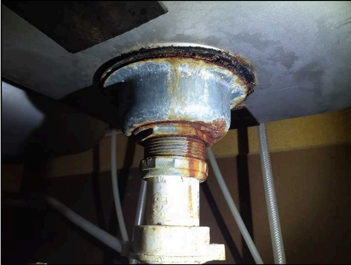
Repair the minor leak at the drain line connection under the basement kitchen sink. Have a plumber examined and repair.
