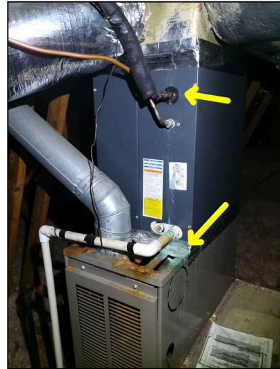
Condensation is dripping from the evaporator coil penetrations when air conditioning was tested. Recommend correction by a qualified HVAC technician.
