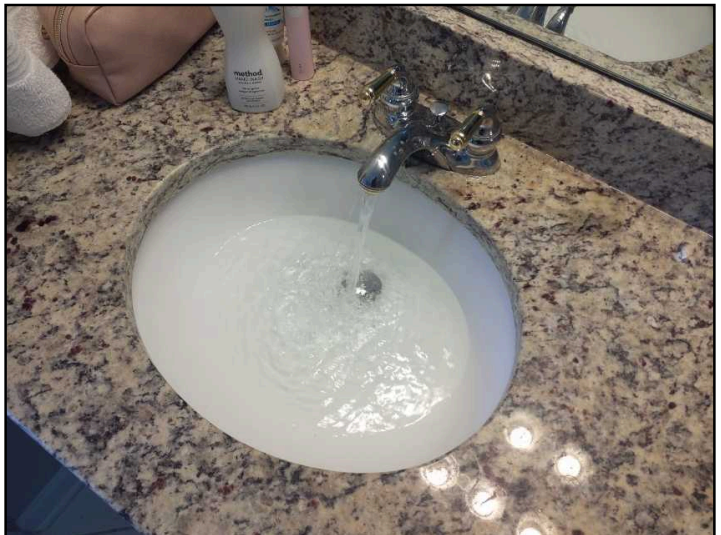
Slow drainage at left sink in master bathroom
