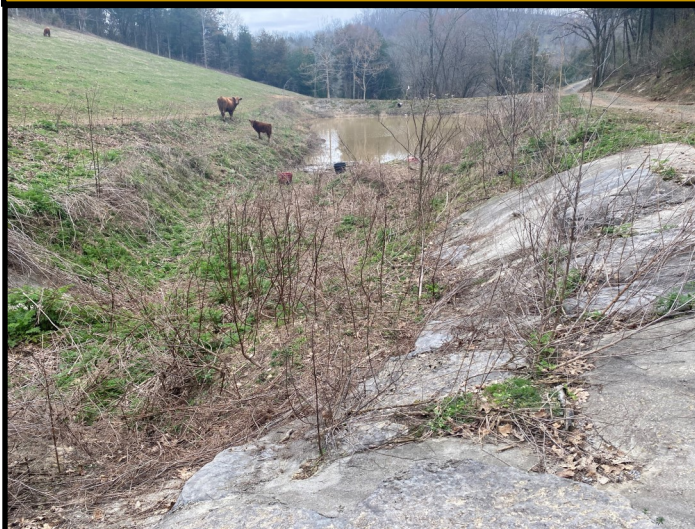
The catch-out pond prior to restart of the project.
