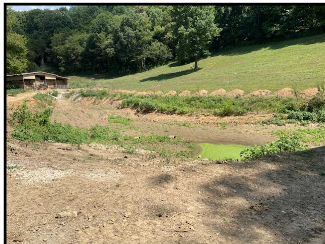
Drained and ready to start repairs.
