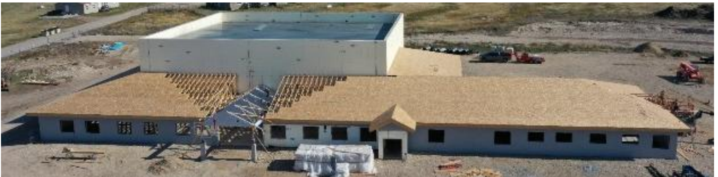
Construction Progress on September 22, 2026. Photo submitted by: Amber Bigby
