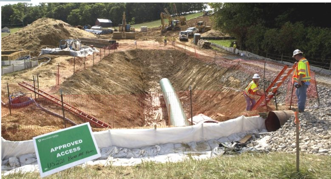
FILE - In this June 22, 2018, file photo, construction crews are boring beneath U.S. 221 in Roanoke County, Va., to make a tunnel through which the Mountain Valley Pipeline will pass under the highway. The U.S. Army Corps of Engineers has suspended a nationwide program used to approve oil and gas pipelines, power lines and other utility work, spurred by a court ruling that industry representatives warn could slow or halt numerous projects over environmental concerns. (Heather Rousseau/The Roanoke Times via AP, File)
