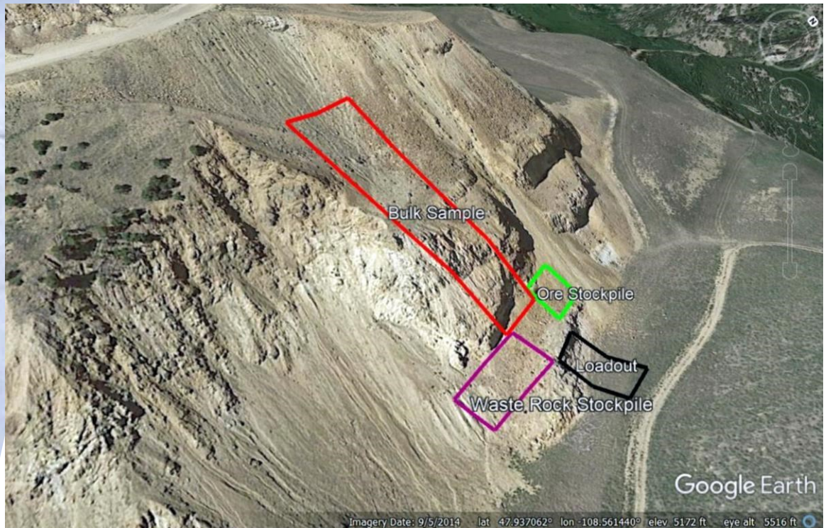
This photo from the Department of Environmental Quality's final environmental assessment shows where the excavation would take place at the old Zortman mine.
