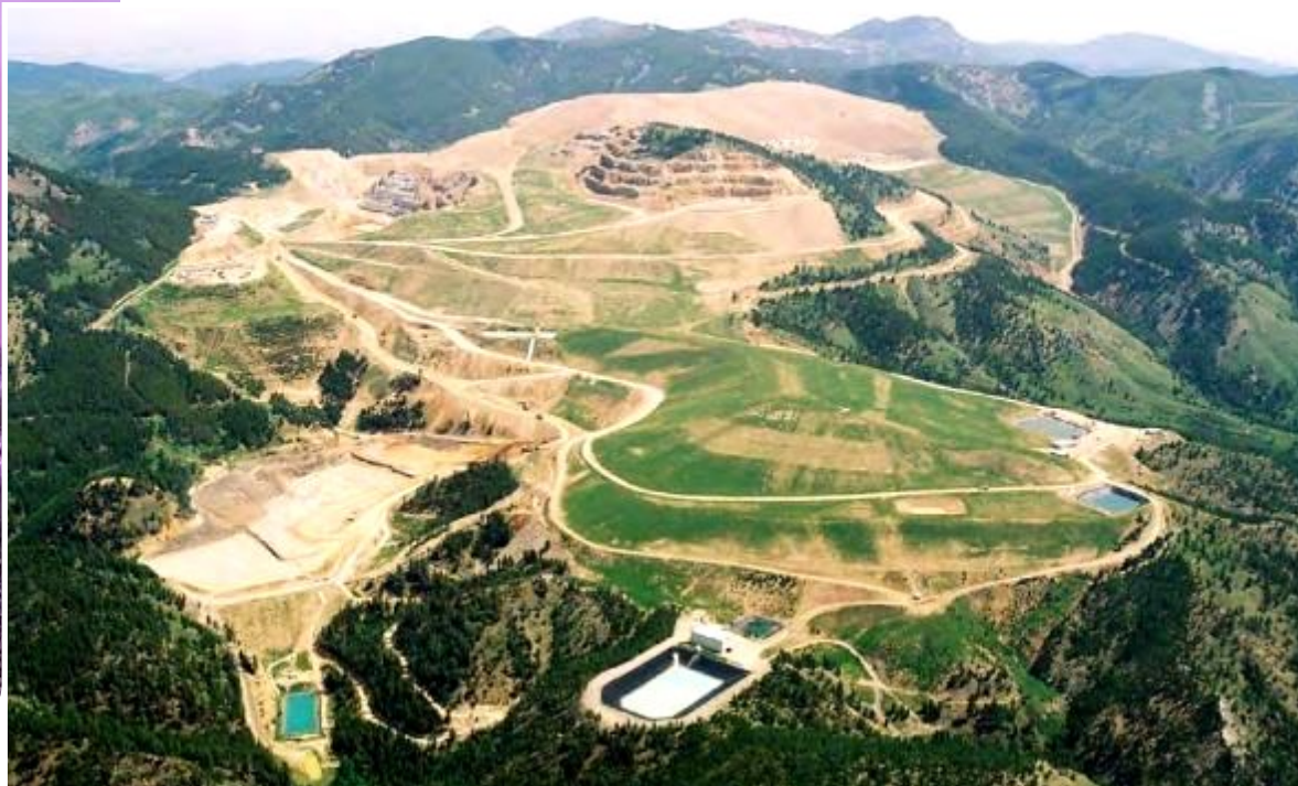
Landusky water treatment facility shown in 2004 (Courtesy Bureau of Land Management).
