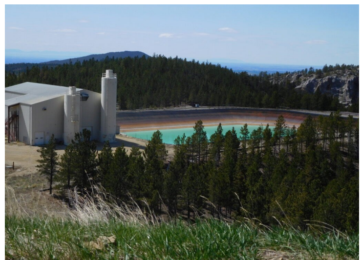
One of two water treatment plants constructed to neutralize acidic water draining from the mine. Because there is no way to stop the exposed rock from generating acidic runoff, mitigation must continue around the clock and “in perpetuity.” Photo by Paul Boyer
