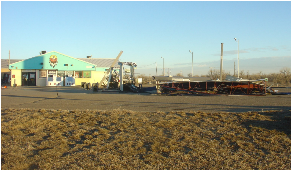
Fort Belknap Kwik Stop wind damage 2.22.2021
