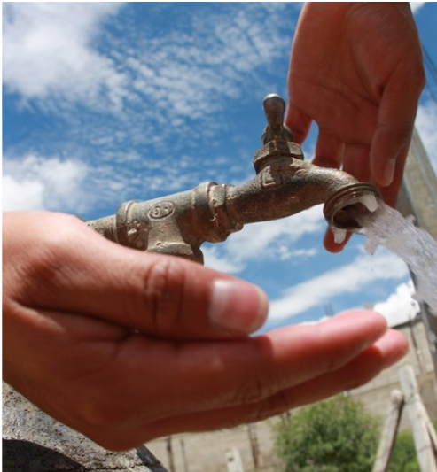
"Drinking water at a side-street water tap" Johannes Roesler, CCBY 2.0
