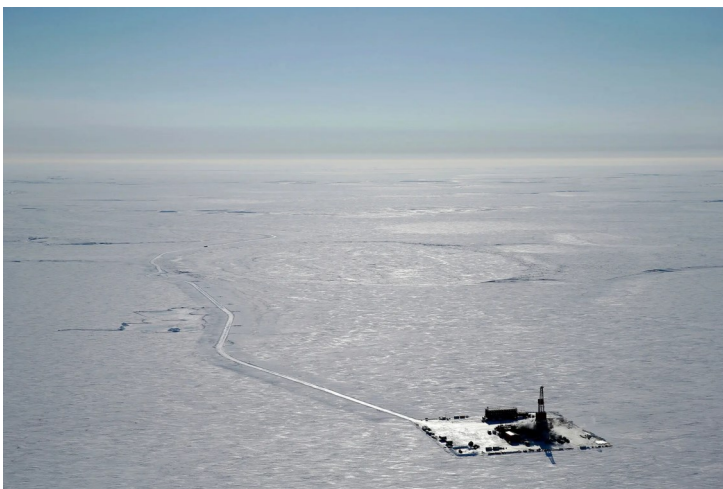
An exploratory ConocoPhillips drilling camp at the proposed site of the Willow oil project on Alaska’s North Slope. Credit...ConocoPhillips, via Associated Press
