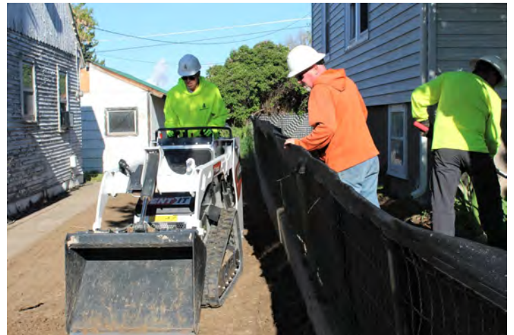
Environmental mitigation crews overseen by the U.S. Environmental Protection Agency have begun work in Black Eagle removing soils contaminated with lead and arsenic.
