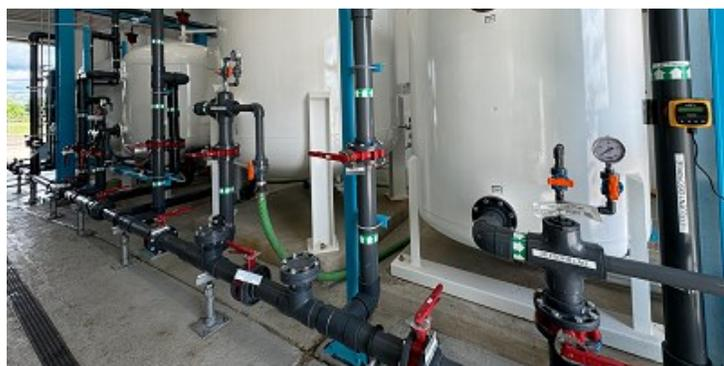
Water filtration system using cyclodextrins at Biddle Air National Guard Base. (Photo courtesy of Cyclopure)
