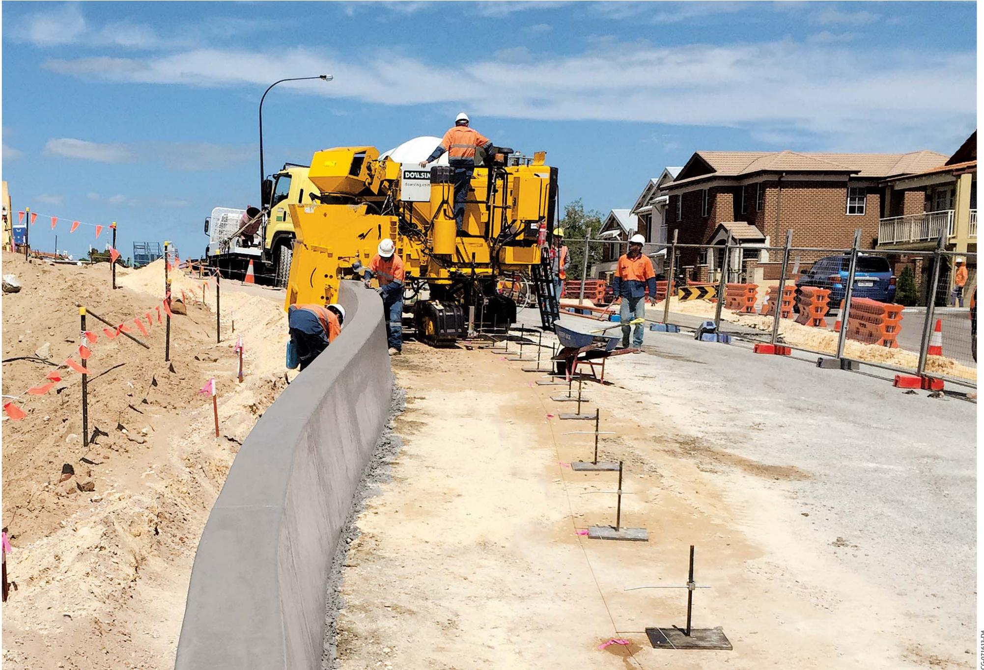
A GT-3600 slipforms variable ranging in height between 34.8 to 50 inches (885 to 1270 mm) on a project in Perth, Australia.
