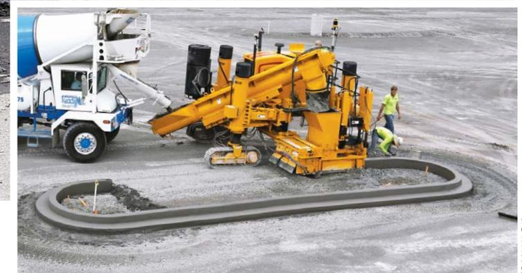
The GT-3600 with 3D machine guidance slipformed radii as tight as 2.5 feet (0.8 m) on this parking lot project. The GT-3600's All-Track Steering, combined with the 3D system's steering algorithms, allow smooth entrances and exits and tighter cornering for tight radii work.
