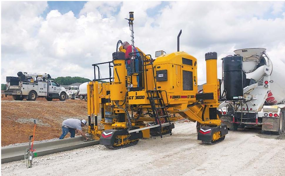
A GOMACO Xtreme GT-3600 slipforms curb and gutter for a new subdivision using 3D machine guidance.
