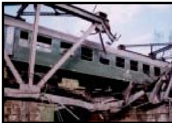
Figure 7-24. Example of a damaged rail transportation system.
