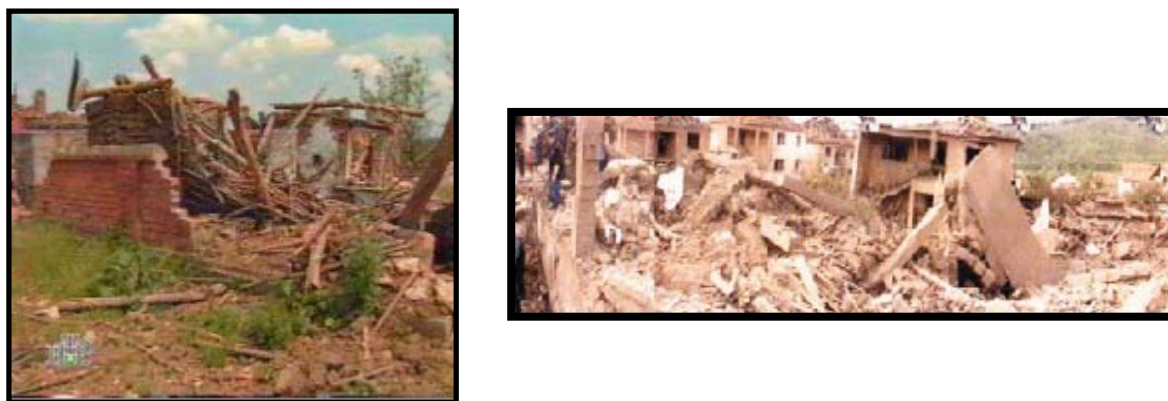
Figure 7-20. Examples of rubble.
